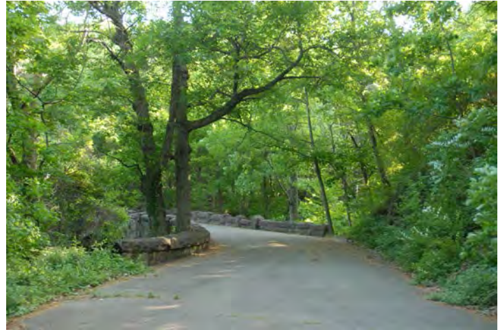
Brownstone bridge adjacent to Trowbridge Drive, East Rock Park, New Haven. Photo by Steve Broker. New Haven SBC.
